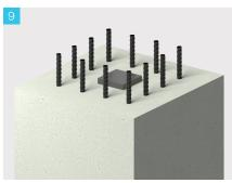
Cast starter bars into the foundation using a suitable template to ensure the location and verticality of the bars.
