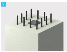
Cast the starter bars into the foundation using a suitable template to ensure the location and verticality of the bars.
