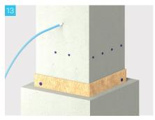
Continue pumping until the grout overflows from the opposite side grouting hose. Then, close the grouting hose holes using a hose caps.
