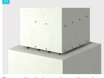
Remove the dust caps. Lower the column onto the starter bars, leaving a small gap to the foundation. Apply any temporary braces as necessary.
