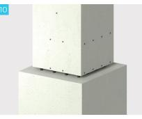
Remove the dust caps. Lower the column onto the starter bars, leaving a small gap to the foundation. Apply any temporary braces as necessary.
