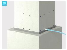
Then, after the grout overflows from the upper grouting hole of the coupler, close the upper and lower hole using a hose cap. Repeat steps 14 and 15 for the remaining couplers.
