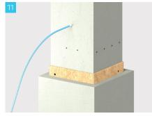
Attach the base formwork to cover the bottom grouting holes and start pumping the grout into the grouting hose.
