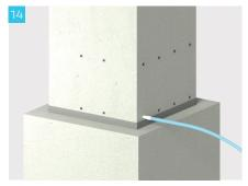
After the base grout is cured, removed the formwork. Start pumping the grout into the lower grouting hole of the coupler.
