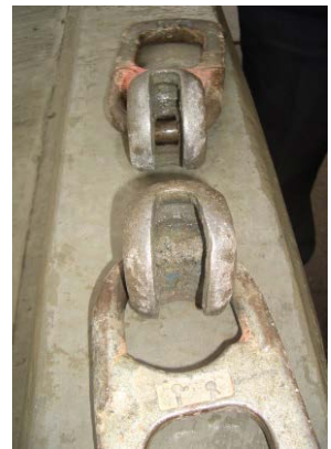
Bent, worn slot
