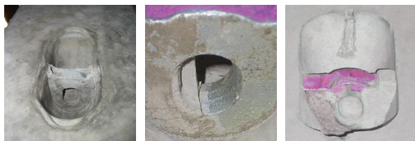
Examples of blocked lifting holes
