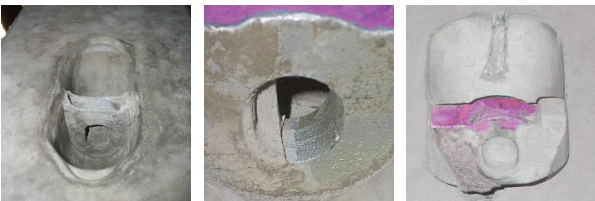
Examples of blocked lifting holes
