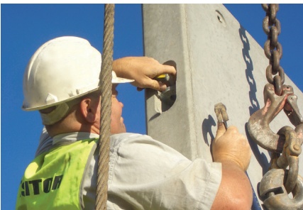
On-site maintenance work required to clean lifting holes
