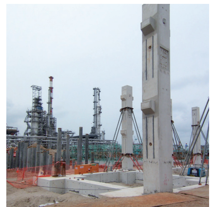
HALFEN HZA DYNAGRIP Channels cast vertically in columns to connect further components.
