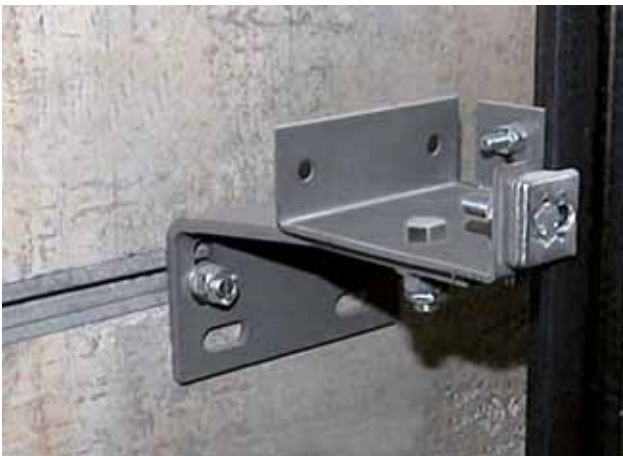
Cast-in channels and bolts
