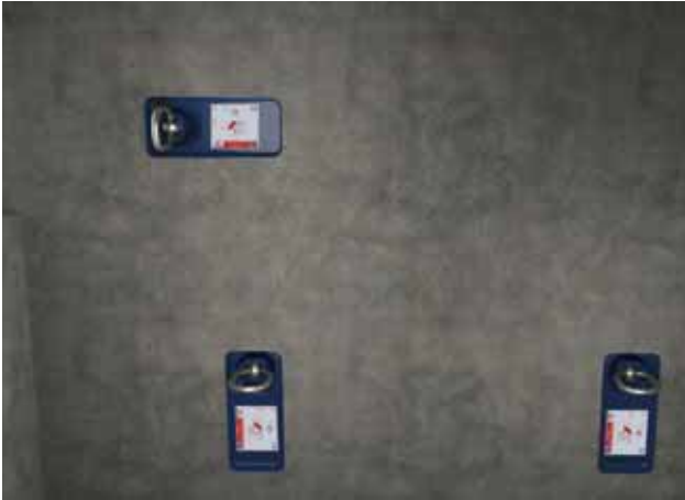
HALFEN HLX-Lift-Box – Cast into the concrete slab at the top of a shaft
