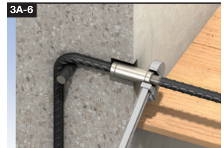
Screw the locknut along the continuation bar to abut the coupler and lock tight with a wrench.
