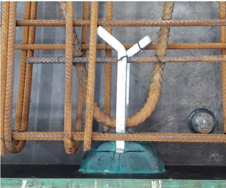
EdjPro Anchor installed with its tension bar. One easy method to ensure the recess and anchor are located hard against the formwork is to push the anchor/recess/tension bar against the sideform and tie the tension bar to the surrounding reinforcement. Fix the reinforcement against the opposite side form to prevent it moving.
