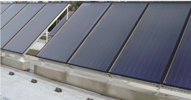
FIXING OF SOLAR PANELS
