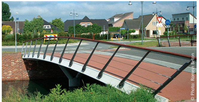
FIXING OF BRIDGE RAILINGS
