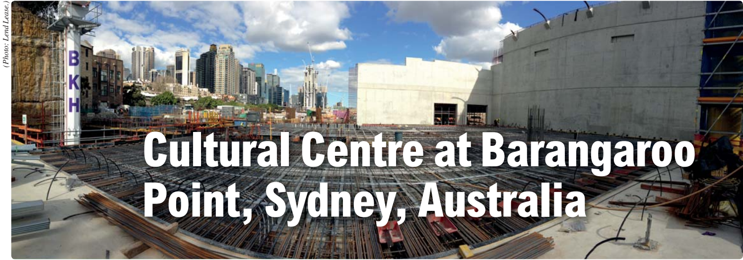
Barangaroo Cultural Centre, post-tensioned suspended floor slab.
