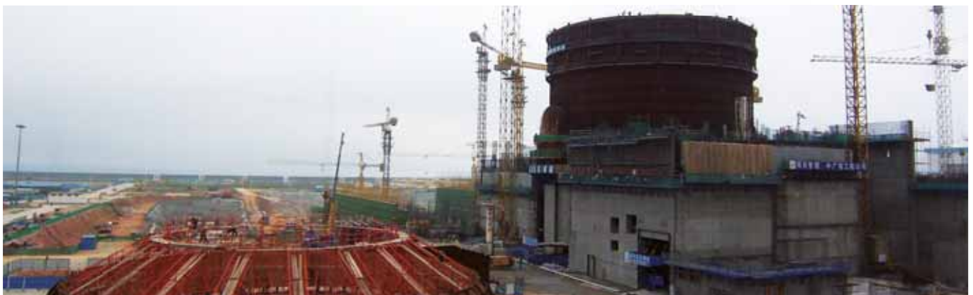
Nuclear power plant under construction
