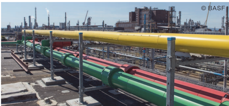
Typical application of the HALFEN Powerclick system
