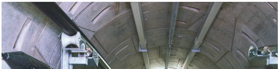
Curved HALFEN Cast-in channels in tunnel segments
