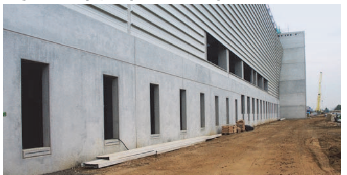
UPS Air Hub, Cologne Bonn Airport, Germany
