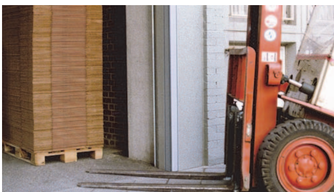
Corner guards in an industrial environment
