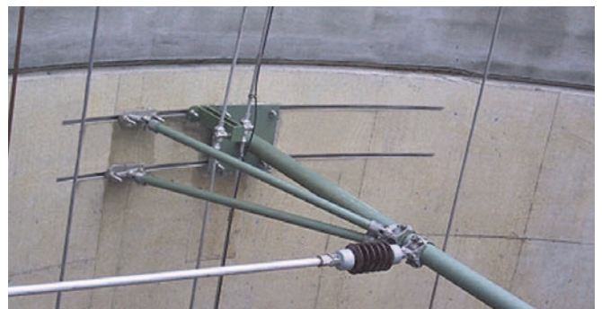
Fixing of overhead cables in railway tunnels
