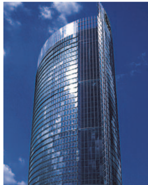
Post office Tower, Bonn
