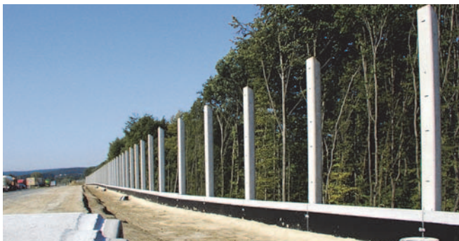
Fixings of noise barriers to concrete posts
