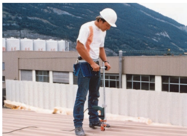
Fixing trapezoidal sheet metal using self-drilling screws
