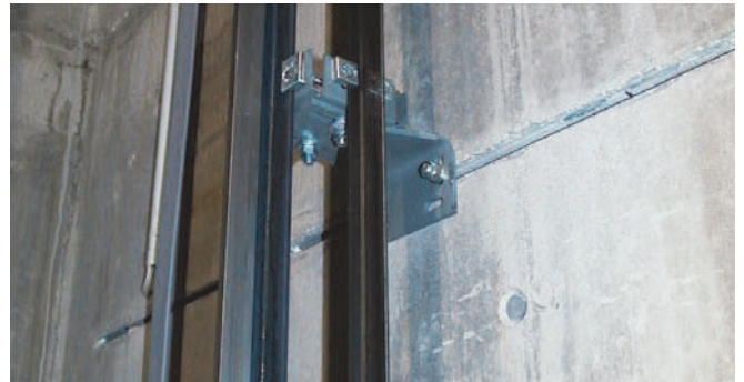
Fixing guide-rails with HALFEN Channels
