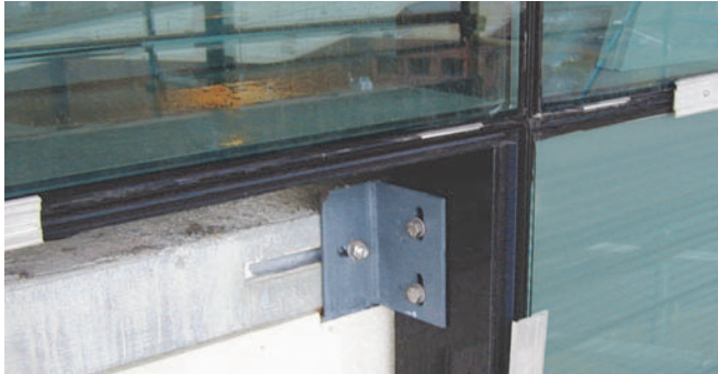
Fixings for curtain wall façades
