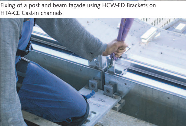
Fixing of a modular façade using HCW-ED Brackets on HTA-CE Cast-in channels
