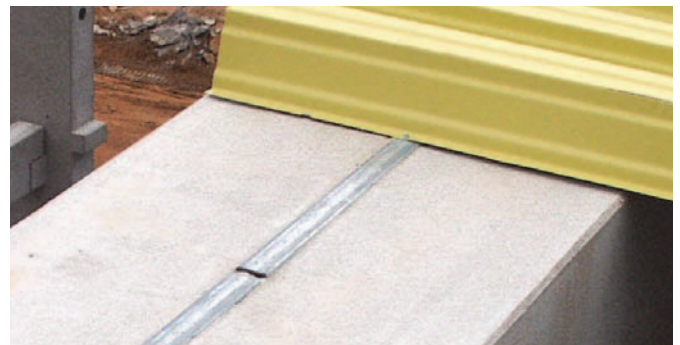
Fixing of trapezoidal sheet metal roof element
