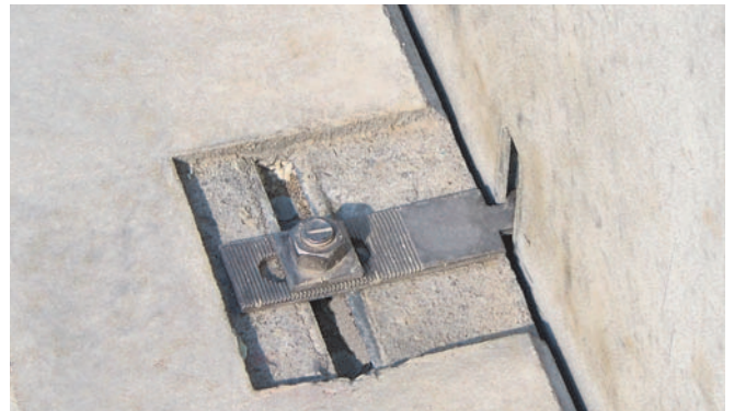
HALFEN HKZ Restraint tie with serrated washer
