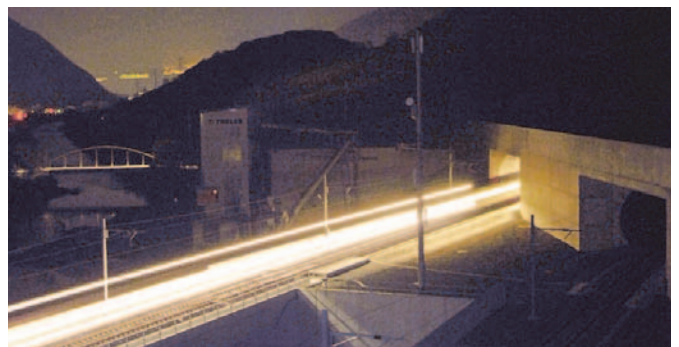
Lötschberg-Base tunnel, Switzerland
