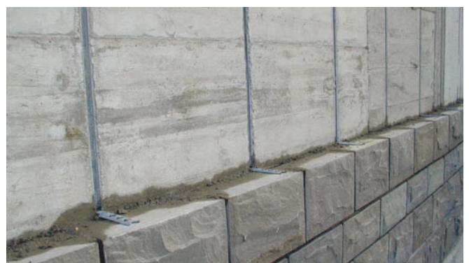
HALFEN ML Brick-tie anchor system
