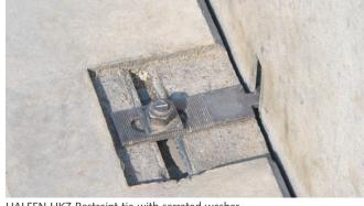
HALFEN HKZ Restraint tie with serrated washer
