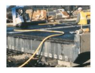
For a perfect fit with the adjacent slab, the endplates were supplied as match-drilled pairs. This guaranteed the precise positioning of 34 bolts at each shear connection. Leviat's dedicated production team ensured all units were delivered to site over a 10 month period to suit the casting yard schedule.
