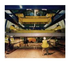
Spanning the river Thames, the Dartford River Crossing forms a vital part of Britain's busiest orbital road, the M25. The Crossing comprises two dual-lane tunnels carrying traffic to the north and a four-lane cable-stayed bridge carrying traffic to the south. Essential remedial work on the East Tunnel required more than 1 kilometre of road deck to be replaced.
