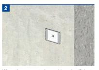
When the concrete has achieved sufficient strength, strike the shuttering. Puncture the label to reveal the hole for the dowel.
