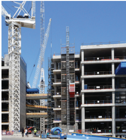
5,000 Lockable dowels were installed on the Royal Children's Hospital, Melbourne, VIC
