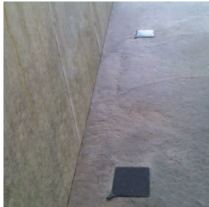
Void formers shown at Slab-to-Wall joint
