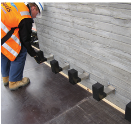
Sleeve pushed over dowel component at core wall
