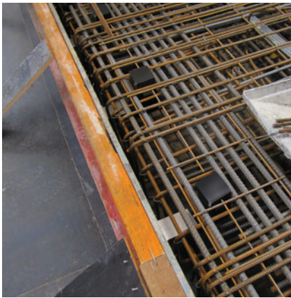
Reinforcement being located around ESDQ-L20 Sleeves
