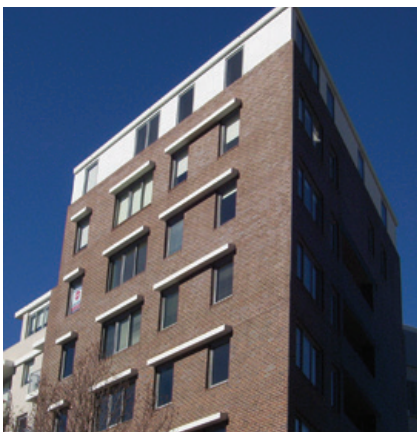
Trinity Apartments, New South Wales
