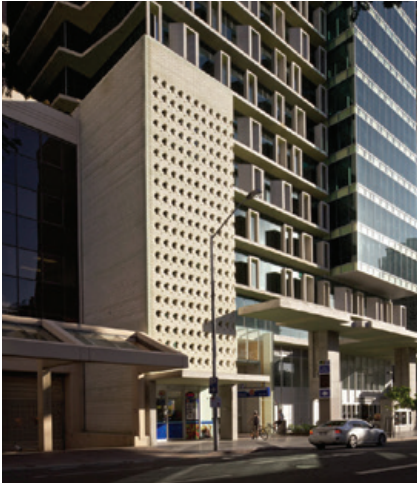
AM60 Building, Brisbane
