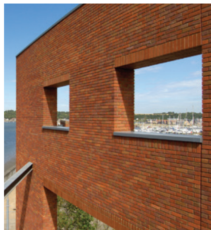
Soffit Support using LDB/S and Soffit Angle
