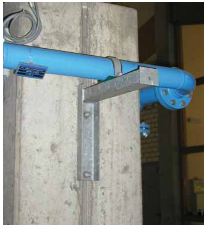
Adjustable pipe support using a cantilever with vertical toothed channel
