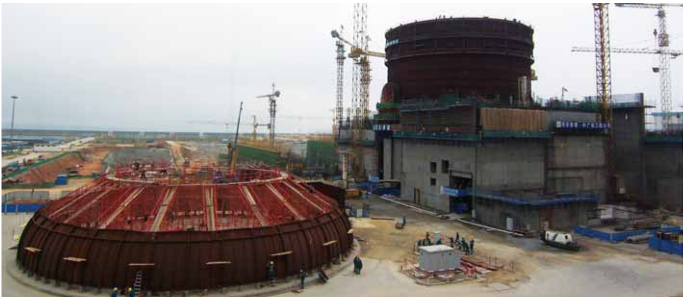
Nuclear power plant under construction
