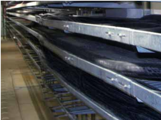
Cable trays accurately levelled by bolting to vertical toothed channels
