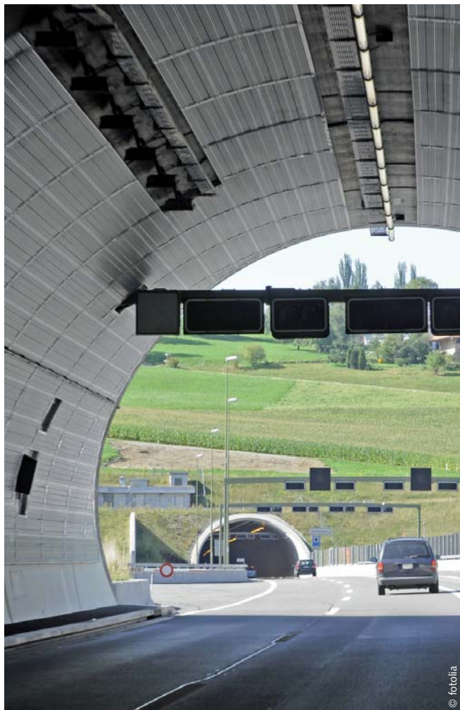
Application sample of HTA-CS 38/17 in HCR quality: highway tunnel
