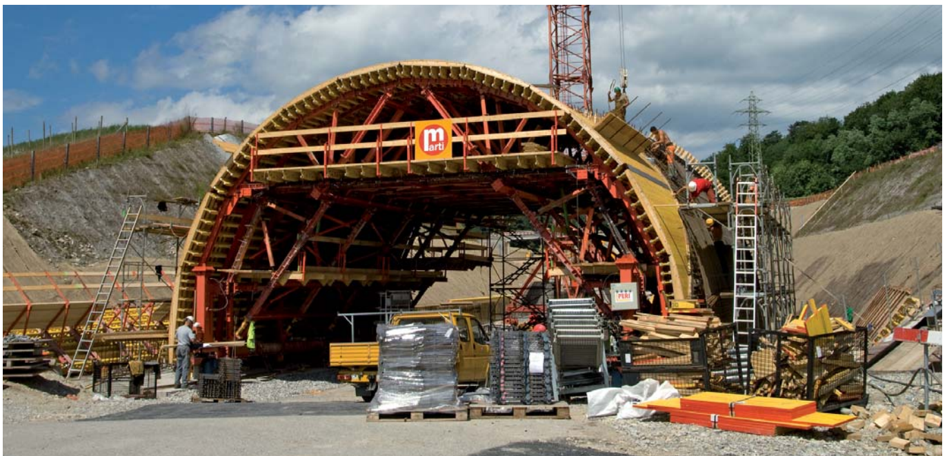
Application sample: HTA-CS on carriage mobile formwork
