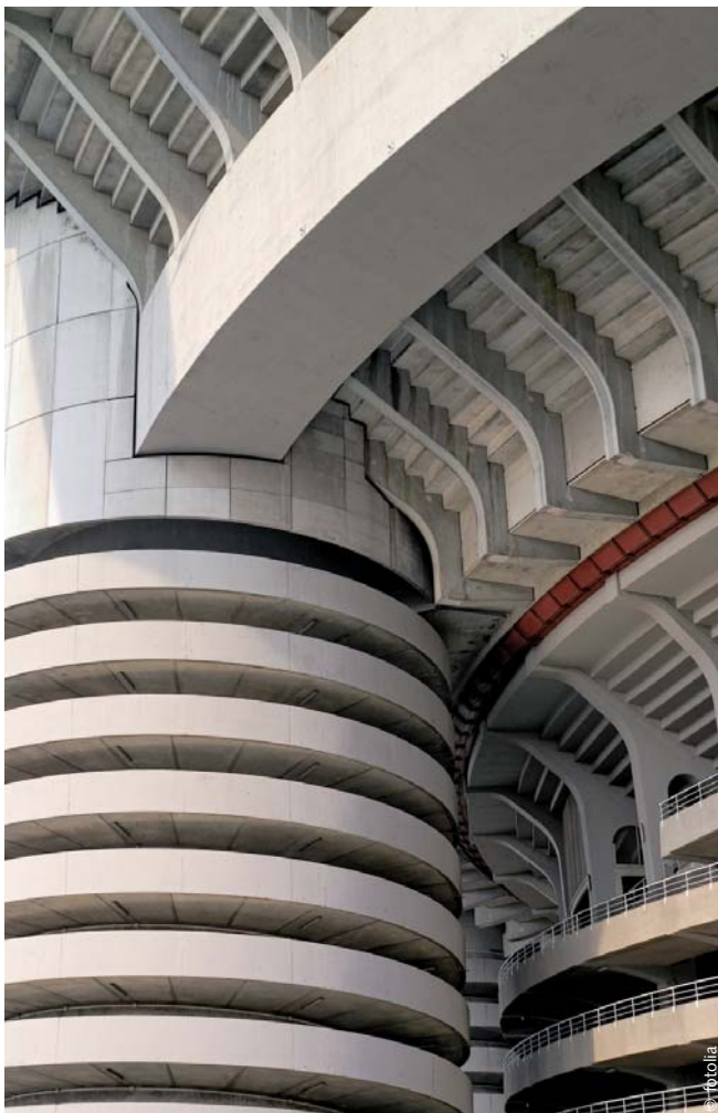
Application sample: HTA-CS in curved concrete building elements
