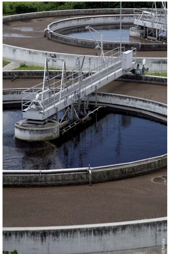
Application sample: HTA-CS in sewage disposal plant
